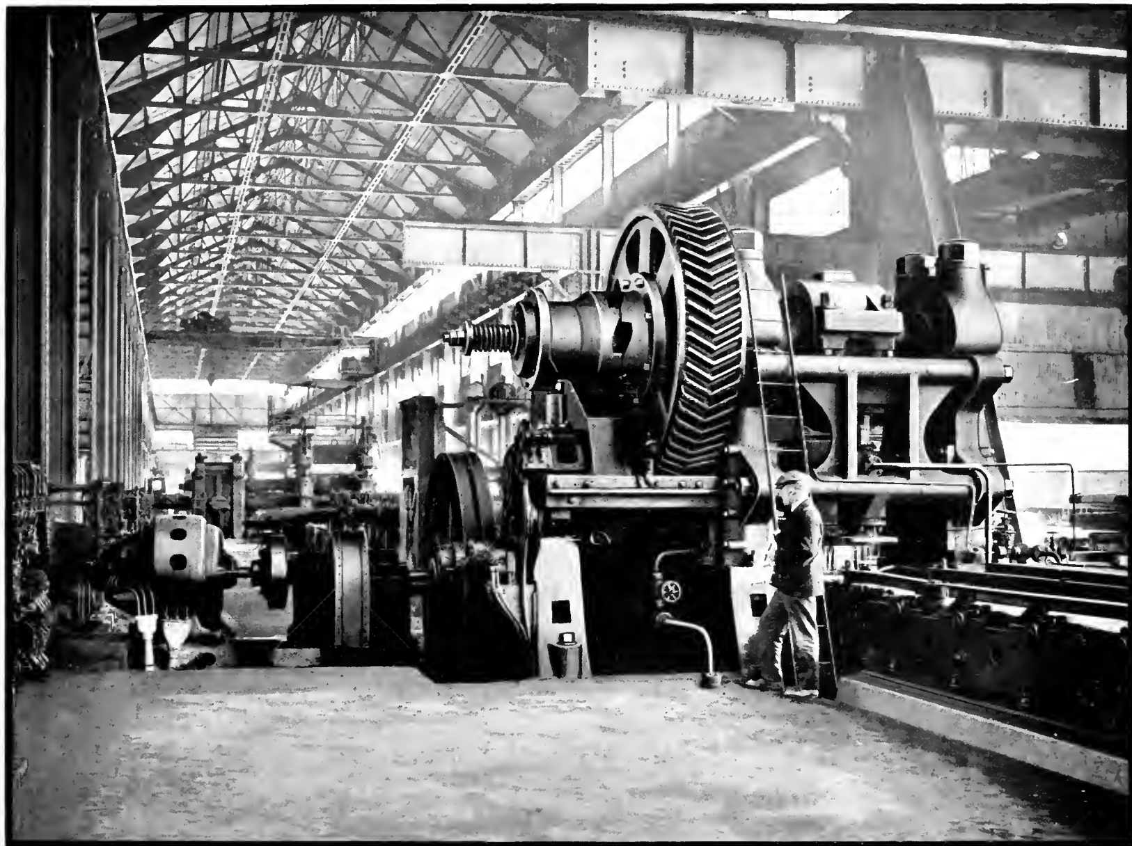
800-Ton Mesta Motor-Driven Bloom Shear Installed at The Central Steel Company
